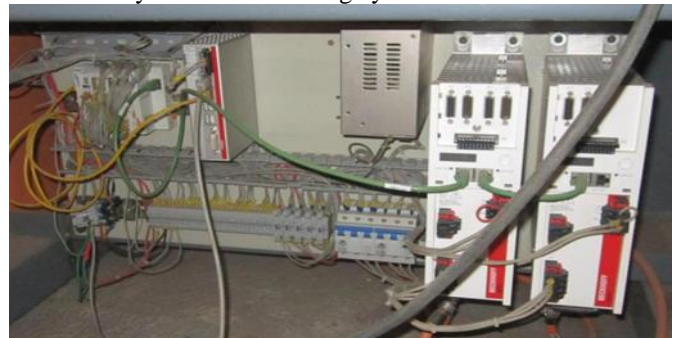
Fig.7 Servo controls and DCIS system
