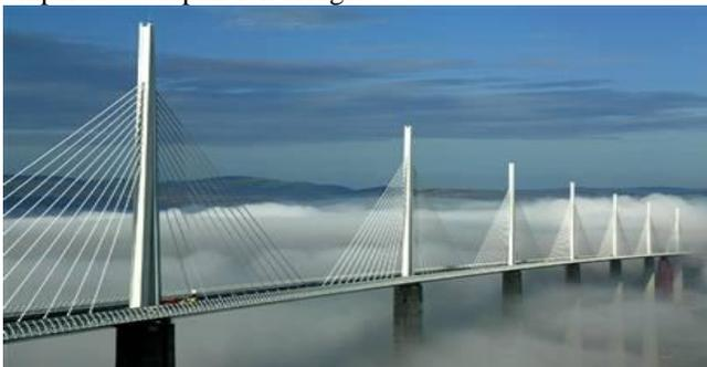
Fig:1.1 A Typical Cable Stayed Bridge
